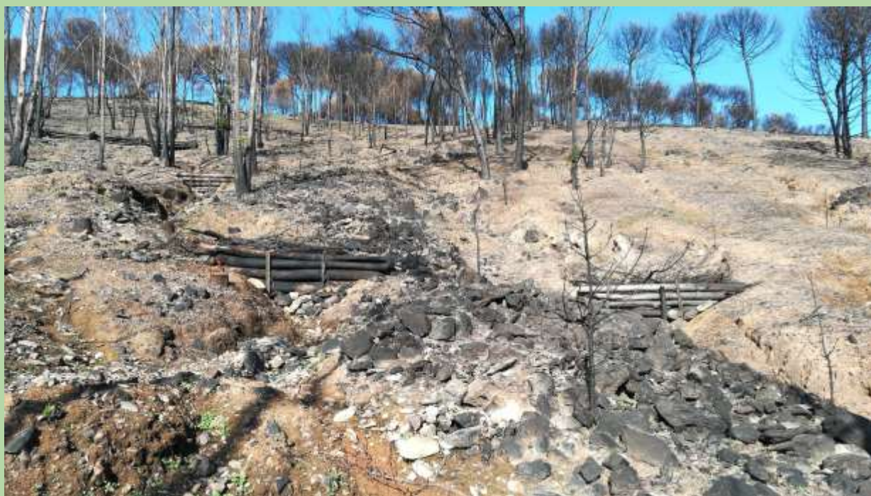
[Check dams (albarradas) on hill slopes - Source: GTA Ingenieria]
