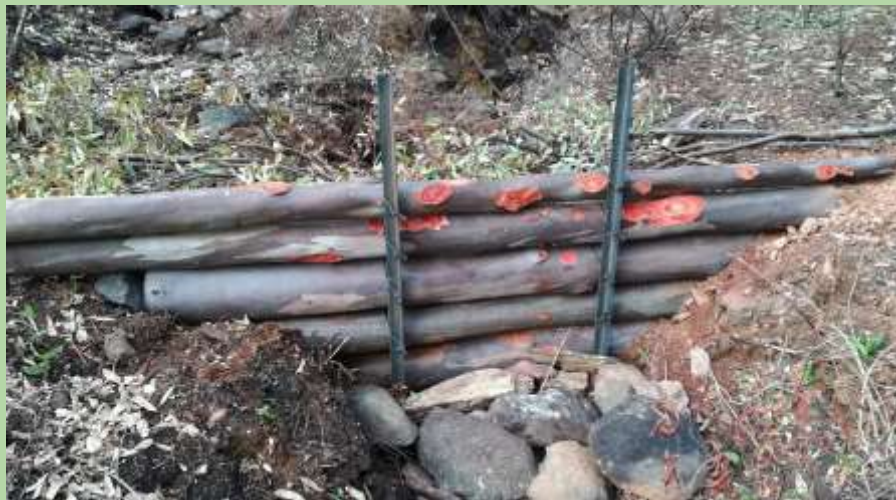
[Eucalyptus-made check dam (albarrada) - Source: GTA Ingenieria]
