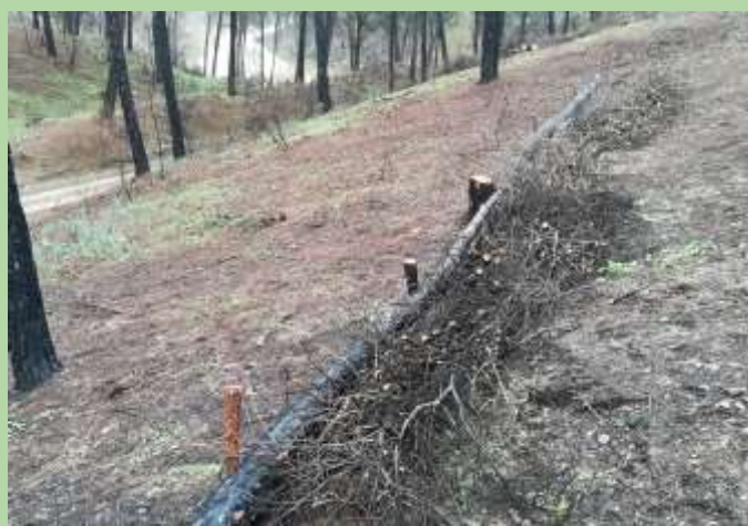
[Shredded biomass residues. Pine-made contour barrier (fajina) - Source: GTA Ingenieria]
