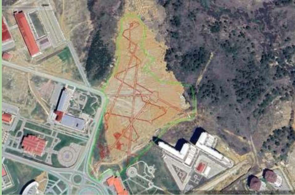
[View of the afforestation work at the Kastamonu University landfill site (4 April 2024) - Source: Kastamonu University]
