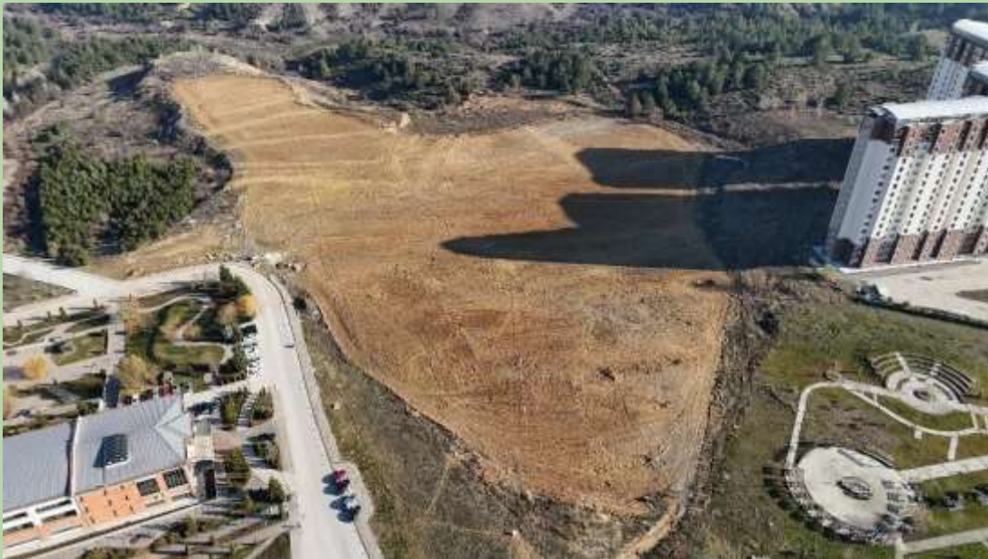
[Kastamonu University landfill site (2023-2024), land preparation, land leveling, soil improvement - Source: Kastamonu University]
