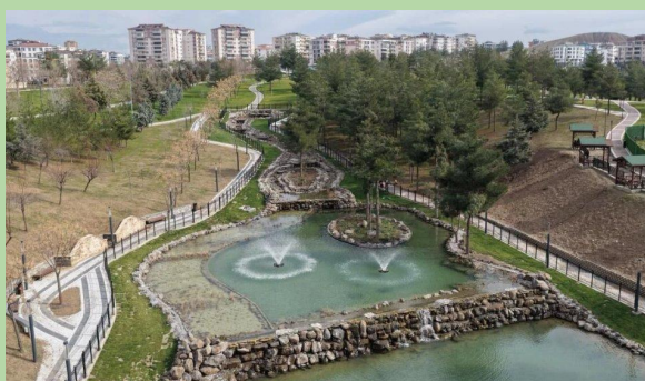
[Completed 2,400 m 2 biological pond (2025): a constructed wetland ecosystem with fountains, cascading waterfall and pine canopy — the ecological core of the park - Source: Batman Municipality]
