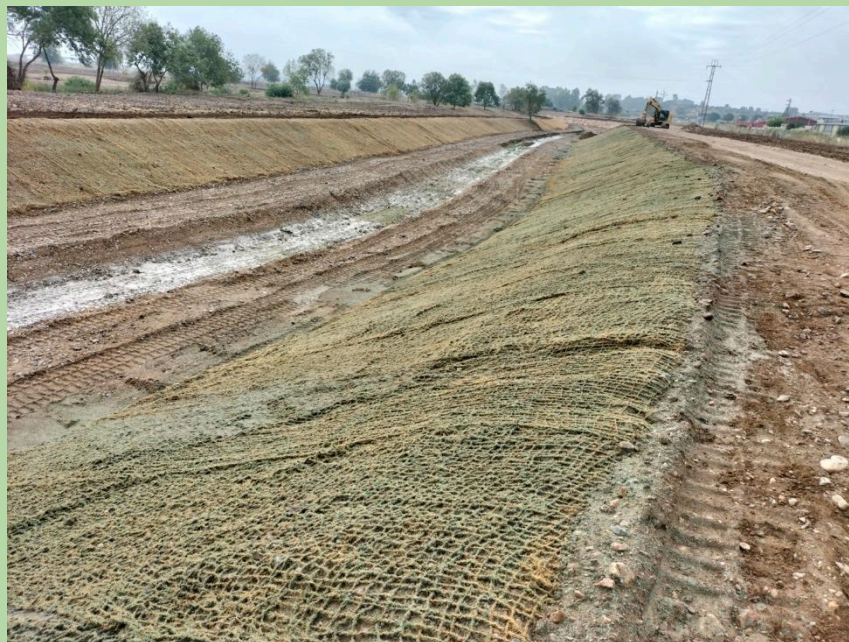
[Slope reduction and installation of a coir erosion-control network for soil retention. Source: Guadiana River Basin Authority - Confederación Hidrográfica del Guadiana]
