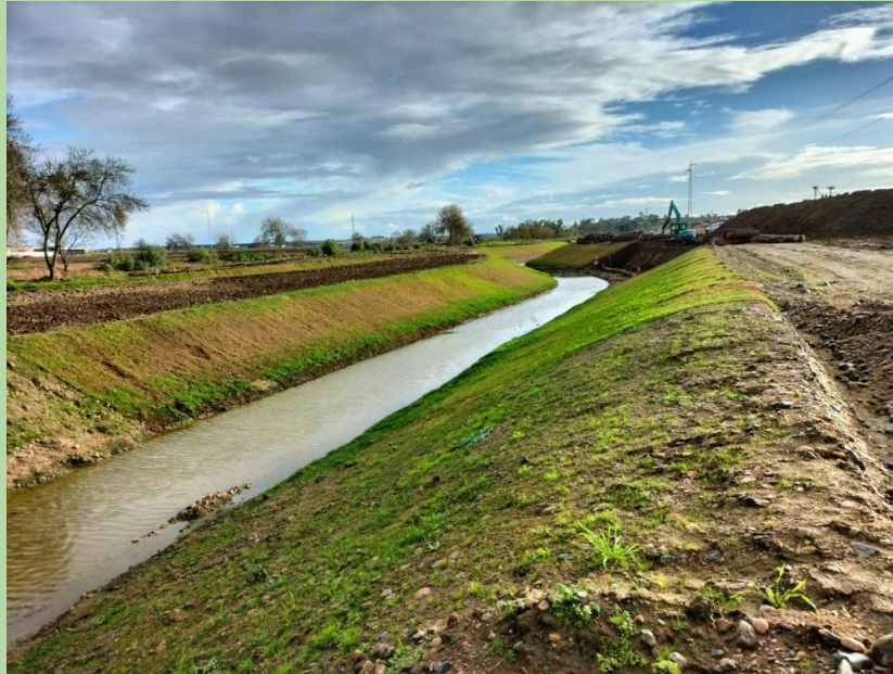
[Hydroseeding for slope stabilization. Source: Guadiana River Basin Authority - Confederación Hidrográfica del Guadiana]
