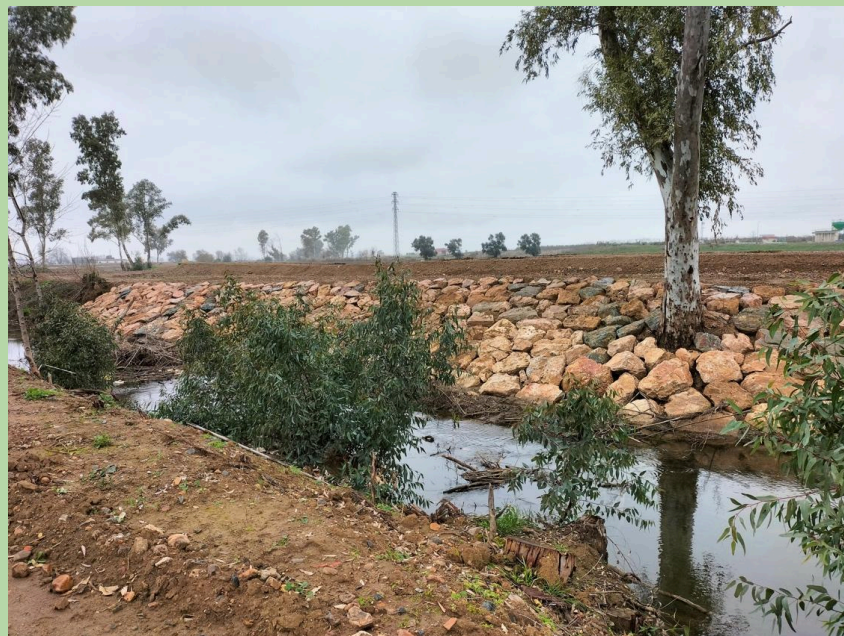
[Protective breakwater construction. Source: Guadiana River Basin Authority - Confederación Hidrográfica del Guadiana]
