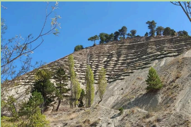
[Shrub-supported (brushwood bundle) terrace constructed on a hillside to reduce surface runoff, trap sediment, and prevent soil erosion. This low-cost, nature-based measure helps stabilize slopes and improve watershed resilience - Source: local units of the project]
