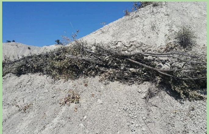
[Shrub-supported (brushwood bundle) terrace constructed on a hillside to reduce surface runoff, trap sediment, and prevent soil erosion. This low-cost, nature-based measure helps stabilize slopes and improve watershed resilience - Source: local units of the project]
