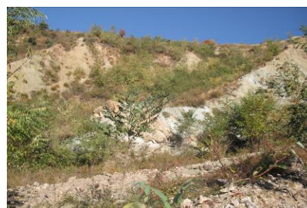
Terrain after intervention
